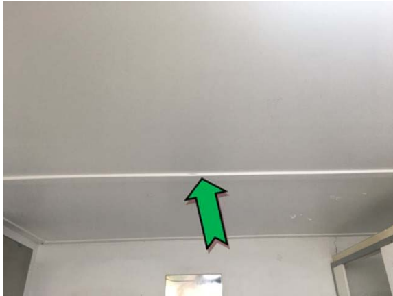
Photo 7. Interior, ladies toilet, ceiling – non asbestos containing fibre cement sheeting.
