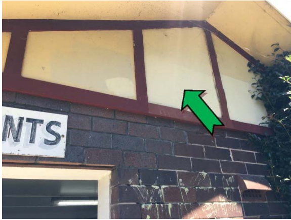
Photo 1. Exterior, male toilets, gable end – non asbestos-containing fibre cement sheeting.
