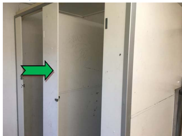
Photo 6. Interior, male toilets, cubicle partition – non asbestos-containing compressed cement sheeting.
